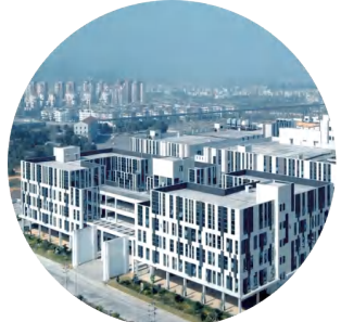
Hubei Production Base
